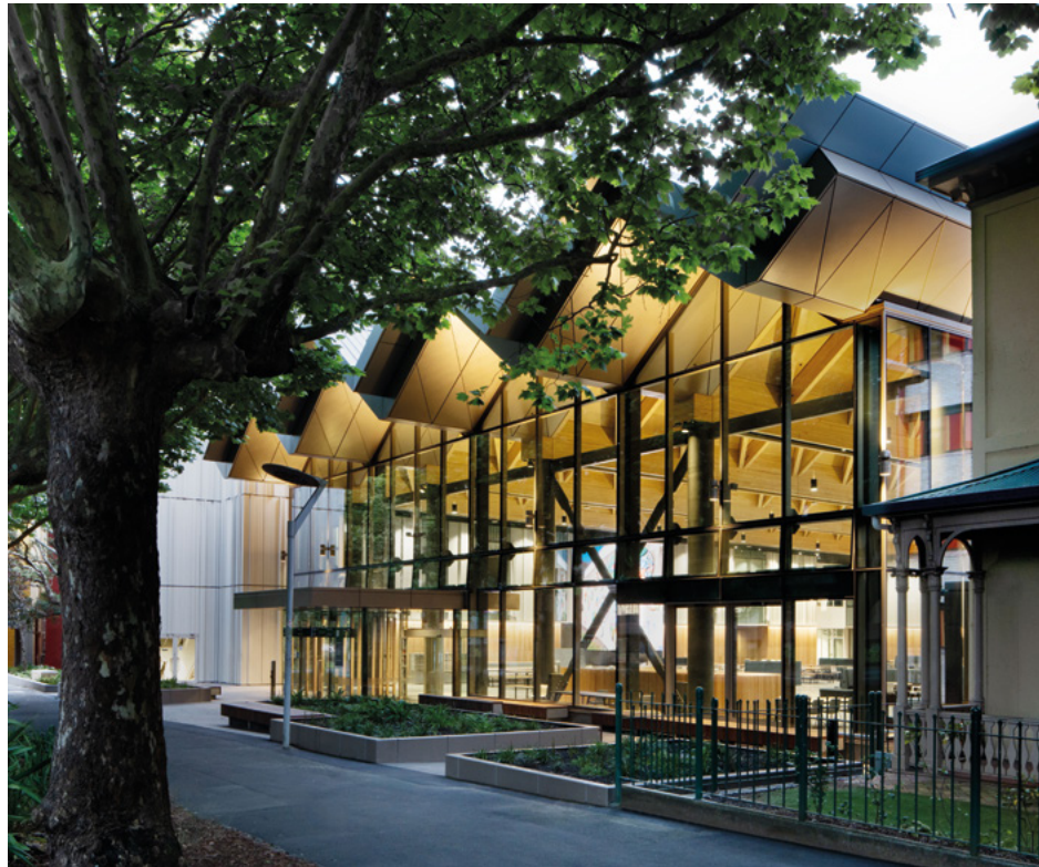
The redevelopment of the University of Auckland's B201 building (submitted by Beca) was the 2026 CIBSE Building Performance Champion
