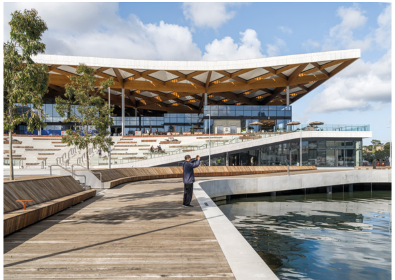
The roof is comprised of 407 prefabricated pyramidal cassettes
