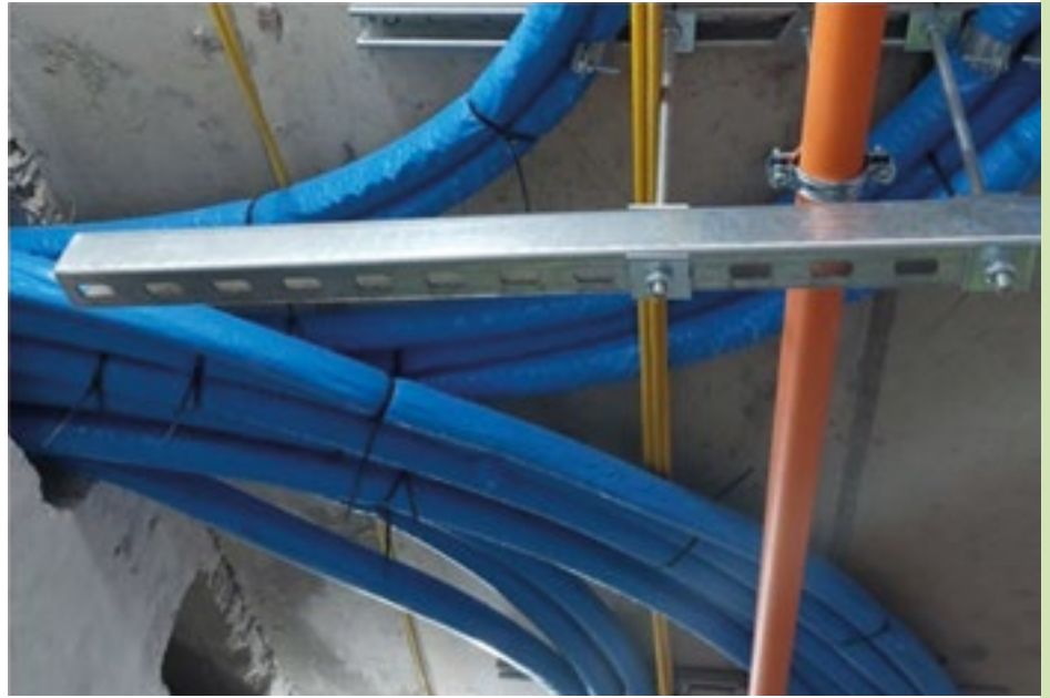
A polyethylene pre-insulated MLCP pipework installation
