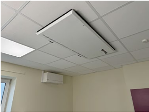
Figure 1: Ceiling-recessed air cleaners use the Coanda effect to distribute air effectively and, at high air-change rates, can achieve very clean room conditions. The units recirculate air after removing viruses, bacteria, mould and any particulates. Recirculating the same air saves energy and reduces carbon impact. This unit has been developed under an NHS-led workstream
