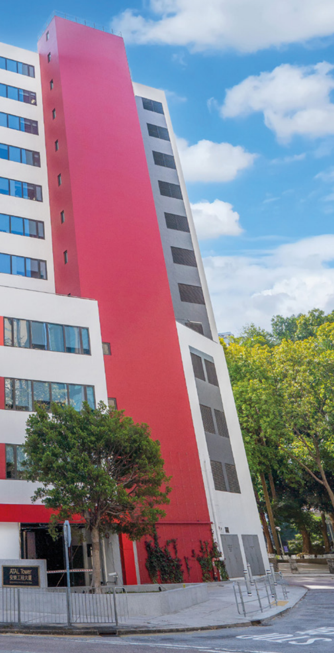
Left: The Atal Tower in Kwai Chung, New Territories, Hong Kong
