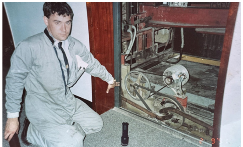
Dave Cooper working on a lift in Carlton House Terrace, London, for Royal Insurance in 1991
