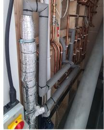
The Modutherm electrode featured before and after insulation
