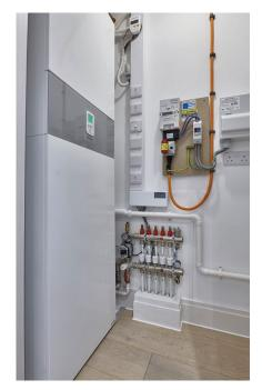
Figure 2: Compact water source heat pump with optional buffer vessel, integrated with a hot–water cylinder feeding an underfloor heating system and supplying domestic hot water (Source: Dimplex)
