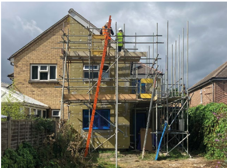
External insulation was installed on the semi-detached Cambridge City Council homes
