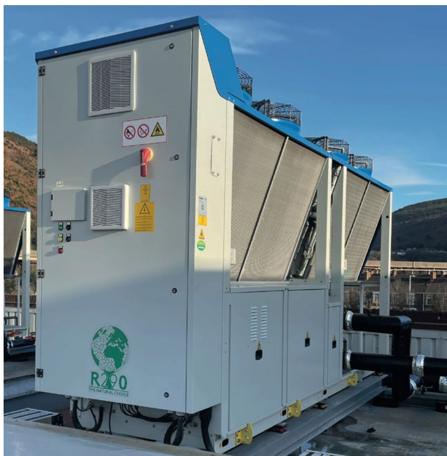
Figure 2: Externally installed air-to-water monobloc heat pumps using propane (R290, A3 refrigerant, GWP ≈ 0.02) supply 40–55°C heating water to AHUs in a UK retail installation achieving a seasonal COP ≈ 4.5 (Source: Swegon)
