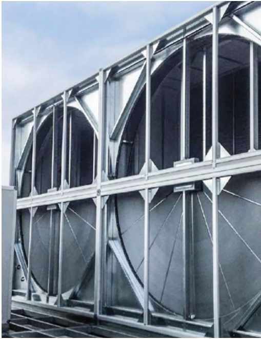
Dedicated fresh-air air handling units incorporate dual heat-recovery wheels
