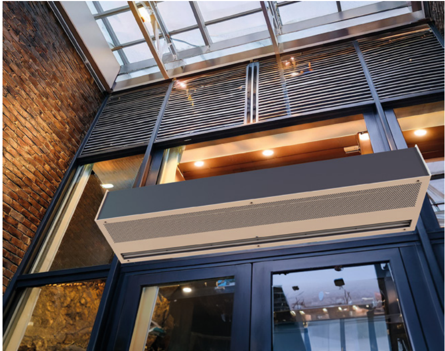
Figure 1: air curtains can be used as a solution to control the dynamic thermal boundary presented by doorways (Source: JS Air Curtains)
