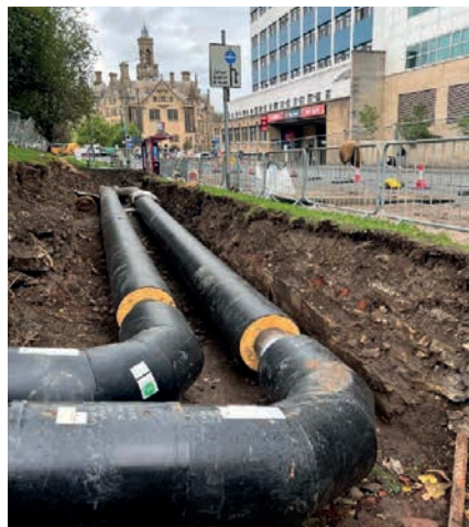
Pipework is being installed beneath the city's streets
