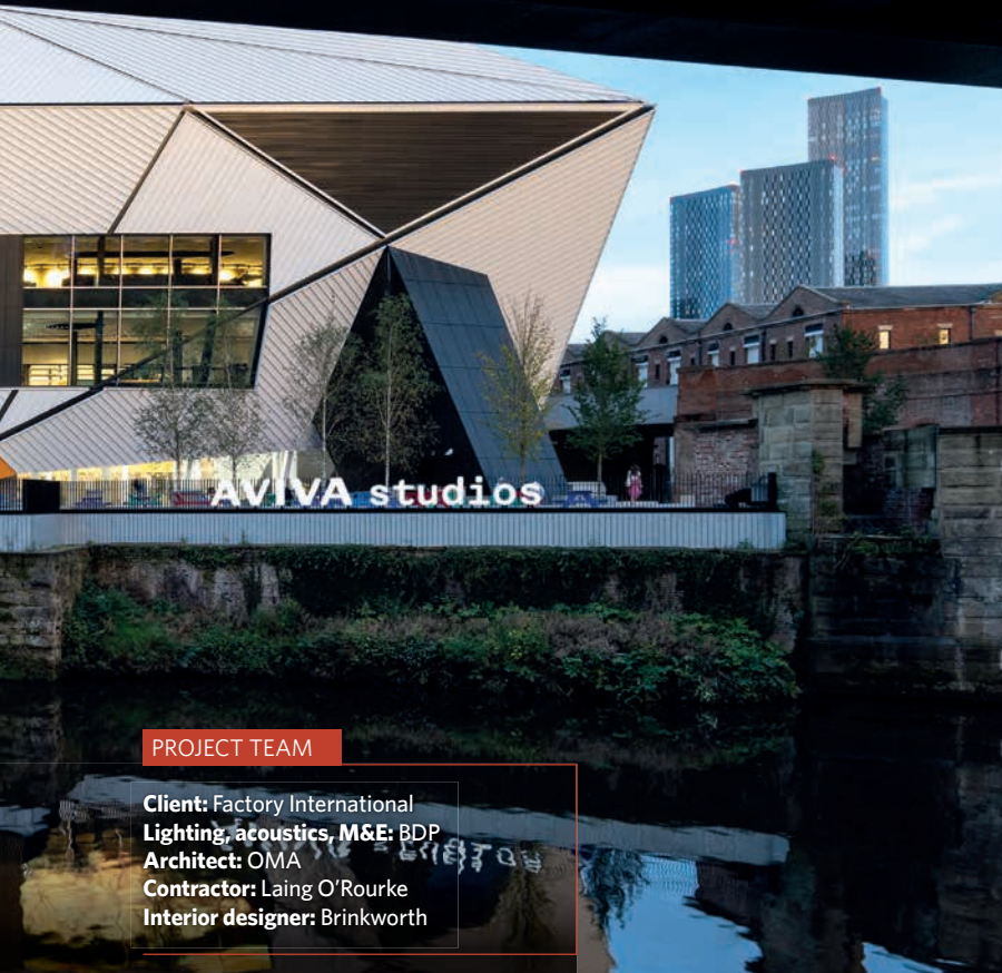
Left: The design of Aviva Studios has opened up public space towards the River Irwell in central Manchester
