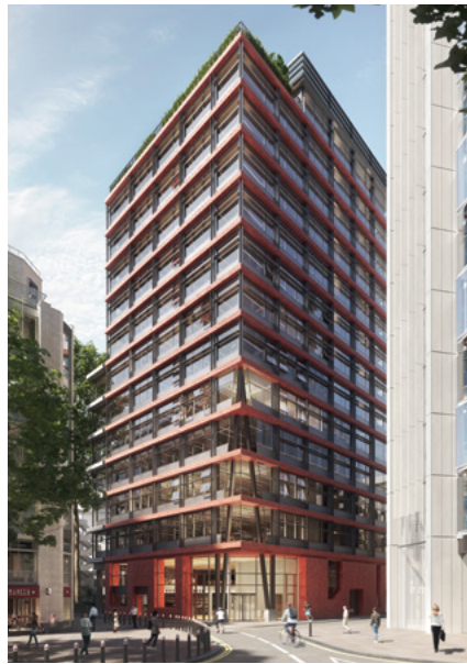
The brise soleil on Edenica is elevation-specific
