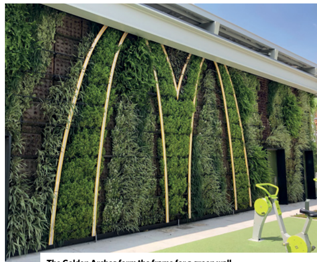
The Golden Arches form the frame for a green wall
