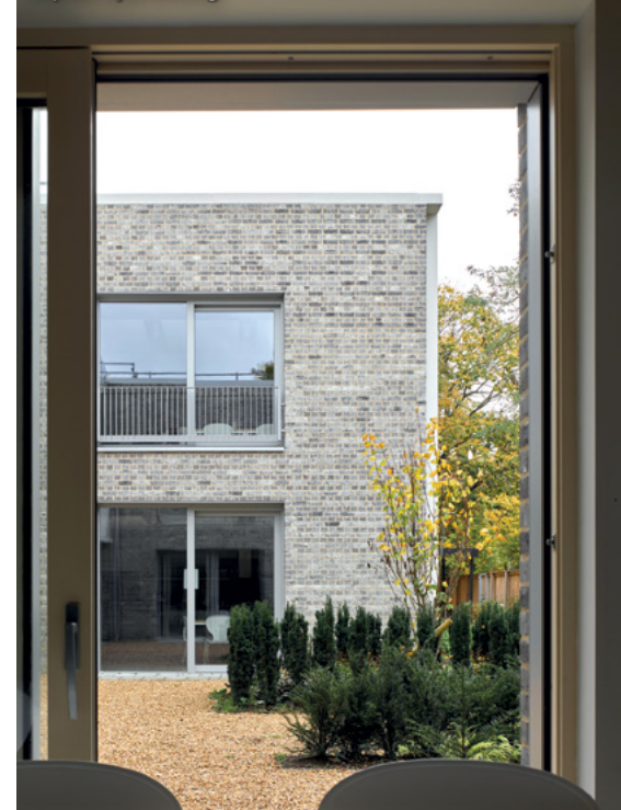
A view from a kitchen in the Stephen Taylor Building
