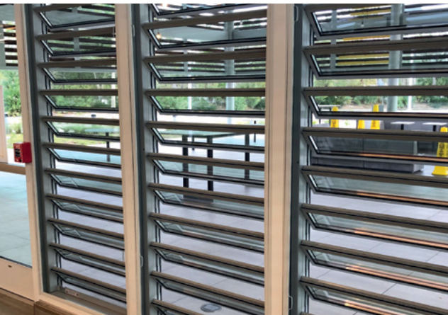
Glass louvres with several safety features provide natural ventilation
