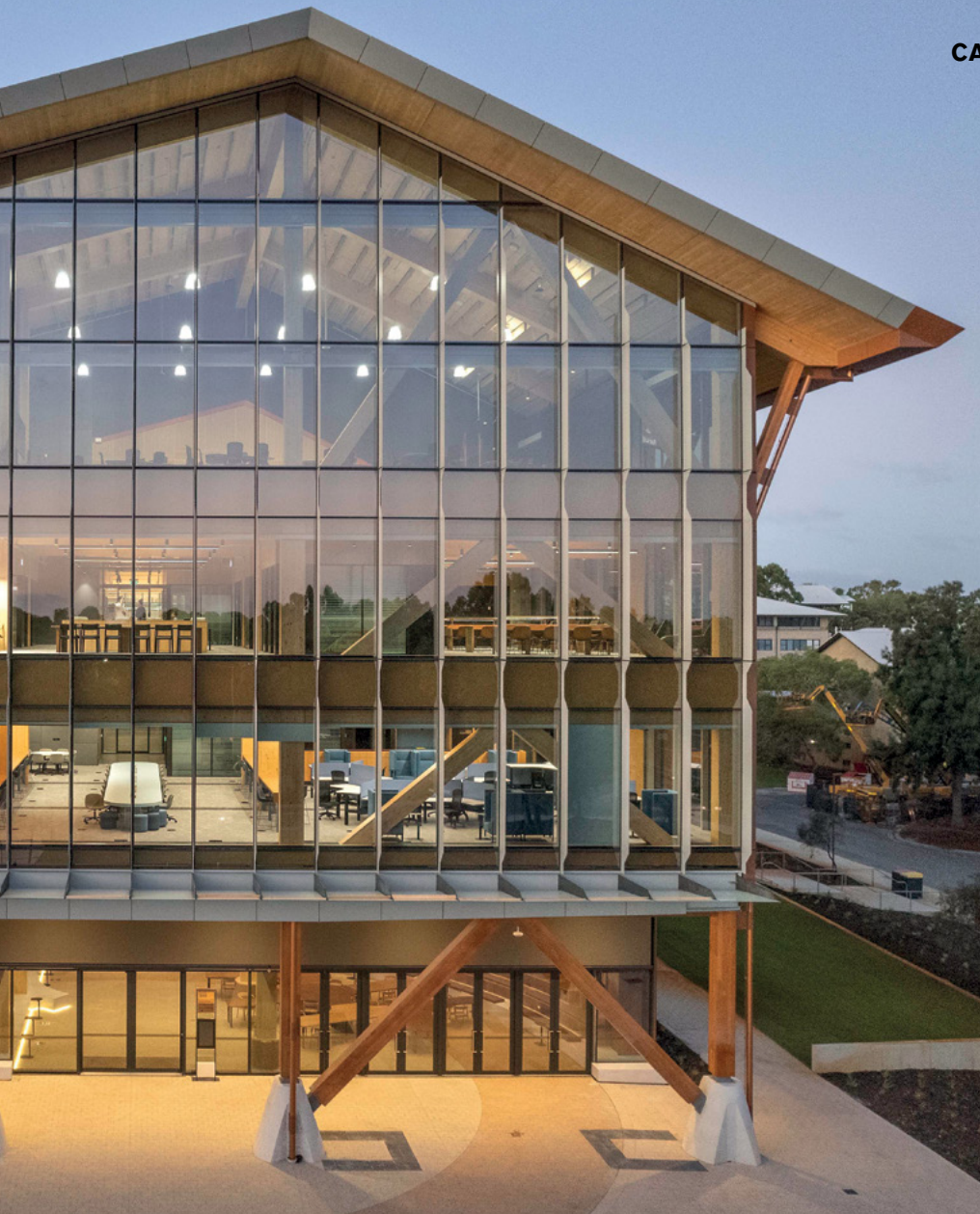
The building is supported on a glulam timber frame
