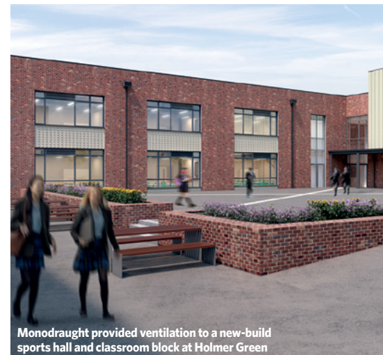
The HVR Zero systems installed in classrooms
