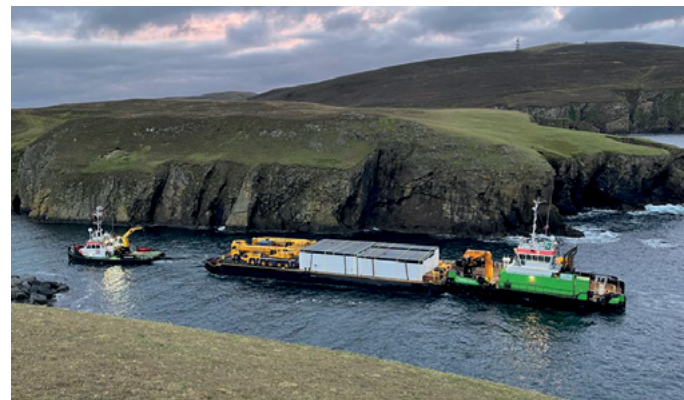
Fully volumetric modular construction was used on a Shetland hotel project
