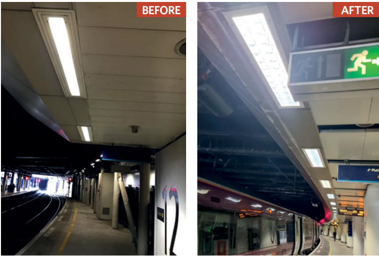
Figure 3: Before and after images of retrofitted platform light at New Street station
