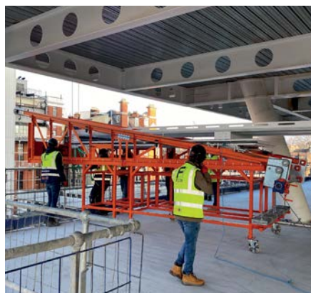
Launch table for unitised façade installation
