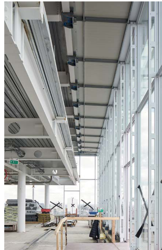
Stick façade at Level 17 restaurant (courtesy of Hufton+Crow)
