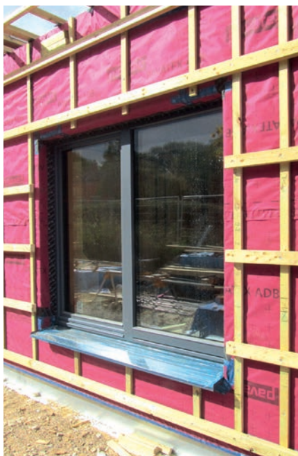
Wind barrier at Larch Corner Passivhaus
