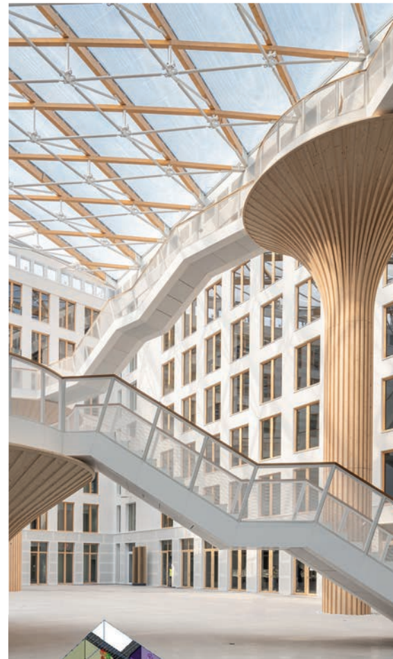
Exposed timber beams on the office floors support the concrete deck of the floor above
