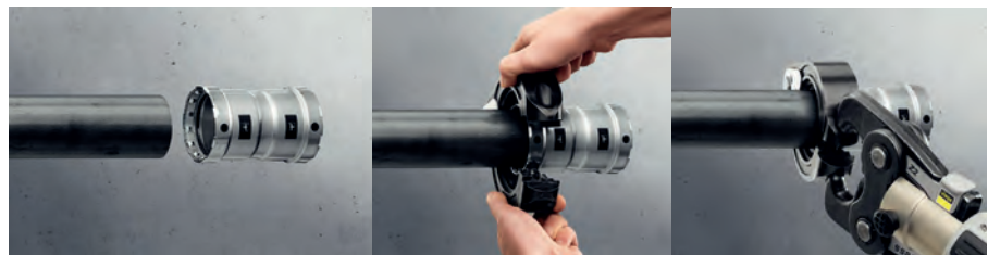
Figure 1: Example of a press connection on a thick-walled carbon steel pipe. The steel pipe is cut to length, cleaned and deburred. The insertion depth is marked and the connector slid on the pipe. The press jaws on the portable machine press the fitting to complete the connection (Source: Viega)
