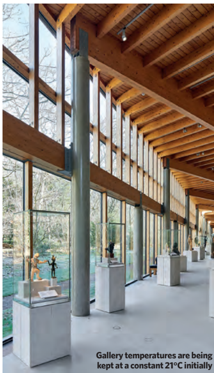
Improvements have reduced the building's peak heat load by about 50% and its cooling demand by at least 20%
