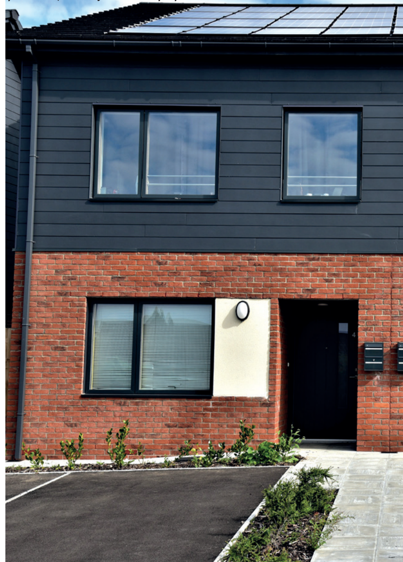
The homes at Rhiw Cefn Gwlad include photovoltaics, PV solar systems and heat pumps
