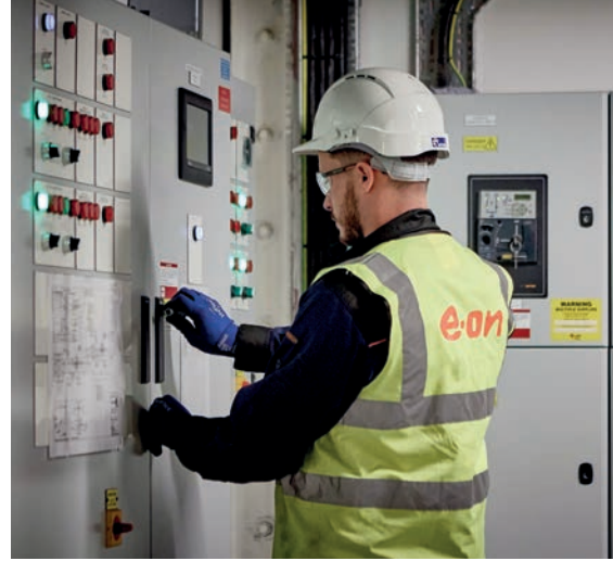
Heat pumps could run on their own without a CHP
