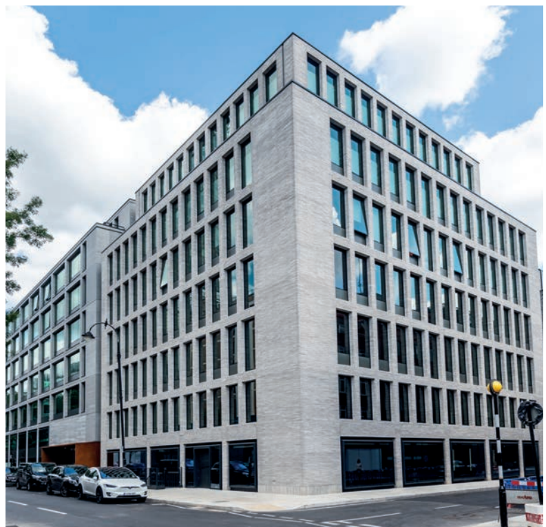
Heat pumps were retrofitted at Arup's 80 Charlotte Street office
