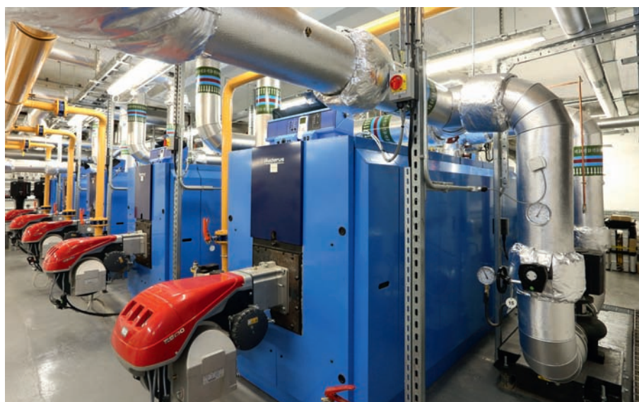
Figure 3: Installed commercial boilers
