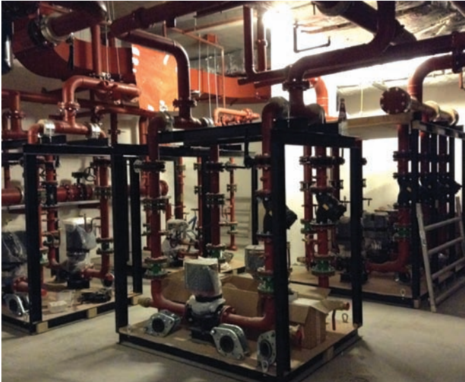
Planning the pump sets installation schedule in BIM avoided trade clashes and minimised access challenges
