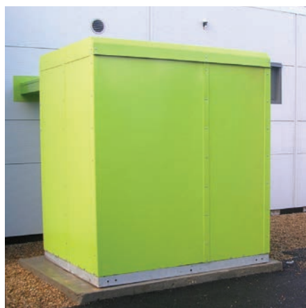
An ICAX Skid controls the transfer of heat to the ground in summer and of heat from the ground in winter
