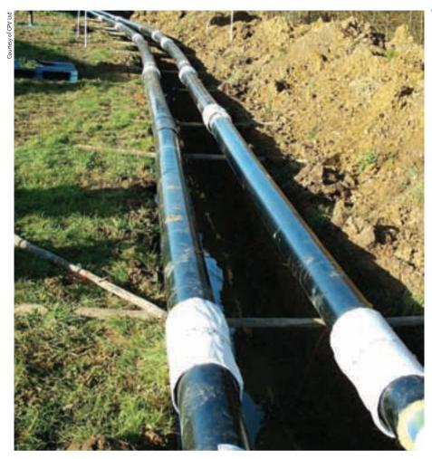
Local district heating systems are increasing around the UK. Here, at the Binton Farm project, at Seale, near Farnham, Surrey, pipes are laid for a new network heating scheme fed by a biomass energy centre
